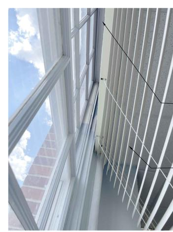
CEILINGS IN SPACES HAVE BEEN LOWERED, AND A BULKHEAD ADDED TO THE WINDOW OPENING AT THE UPPER TWO PANES OF GLASS. (TYP IN 1ST FLOOR WINDOWS)
